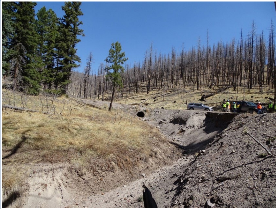
36"x 40' CMP Culvert
